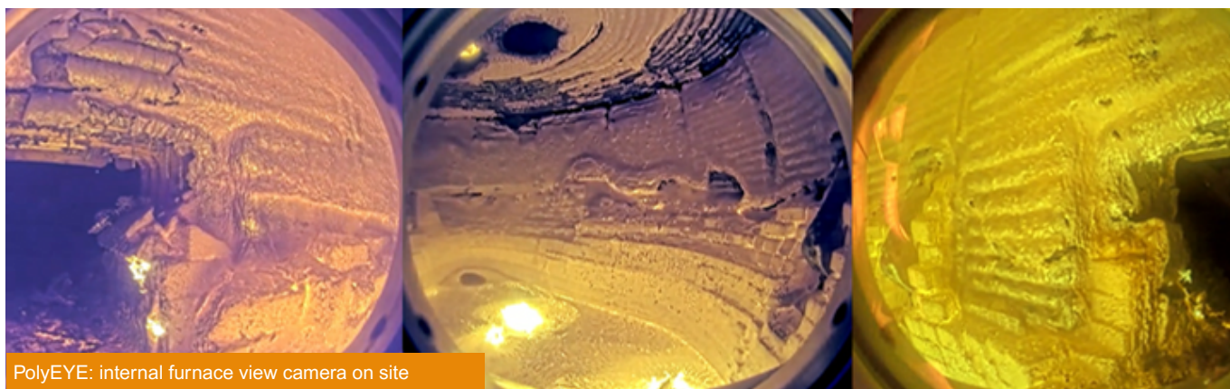
PolyEYE: internal furnace view camera
